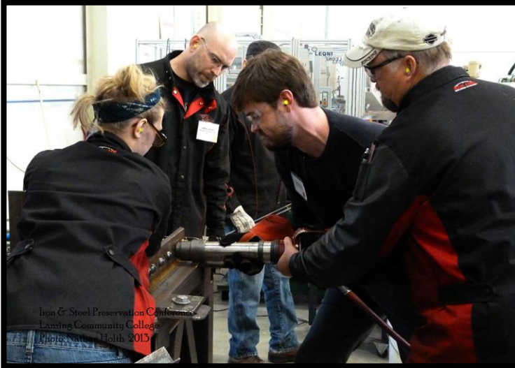
Participant drives rivets with a field riveting hammer, assisted by LCC lab tech Jenna Lone (left, with holder-on) and LCC instructor Roger Morrison (right)
