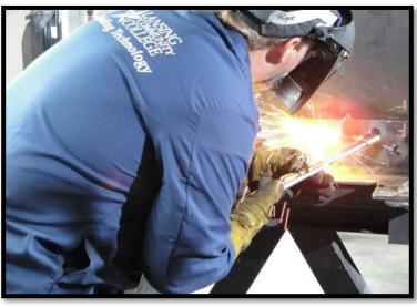
Roger Morrison removes rivets with a oxyacetylene gouging tip
