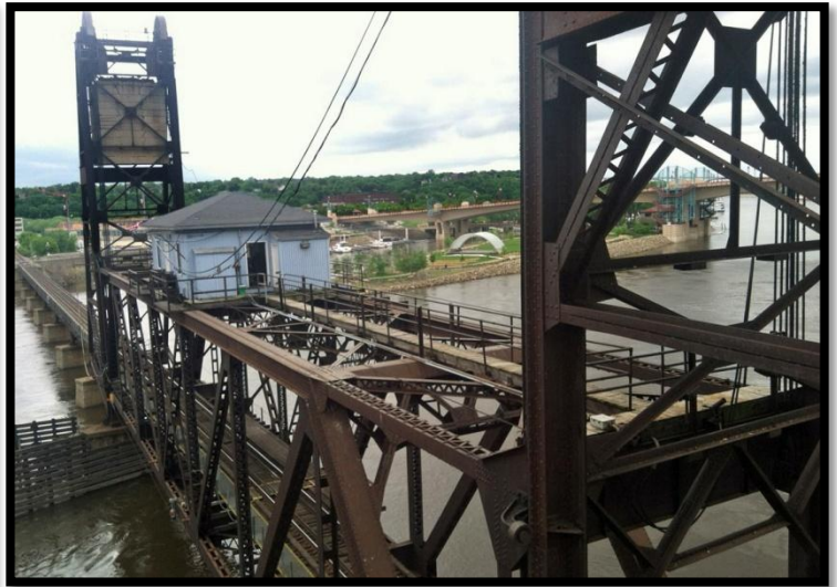
Chicago Great Western Railway Vertical Lift Bridge. Tour participants saw the lift bridge in operation to allow the riverboat to pass underneath.
