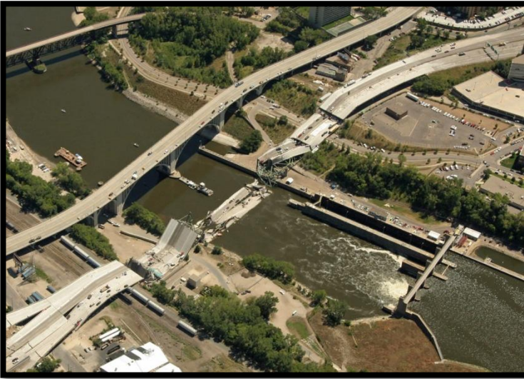
August 1, 2007, the I-35W bridge near Minneapolis collapsed into the Mississippi River. One possible cause for the collapse was undersized gusset plates connecting sections of the bridge trusses. (Source MN Department of Transportation)
