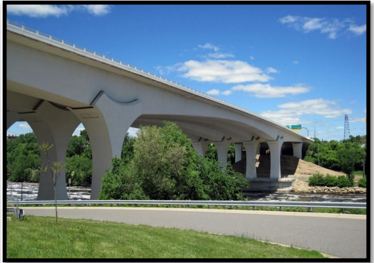
Late fall of 2007 construction began on a new I-35W Saint Anthony Falls Bridge, completed December 24, 2008. Flatiron Contractors and Manson Construction built the bridge. Linda Figg, CEO of Figg Engineering Group, was lead bridge designer.
