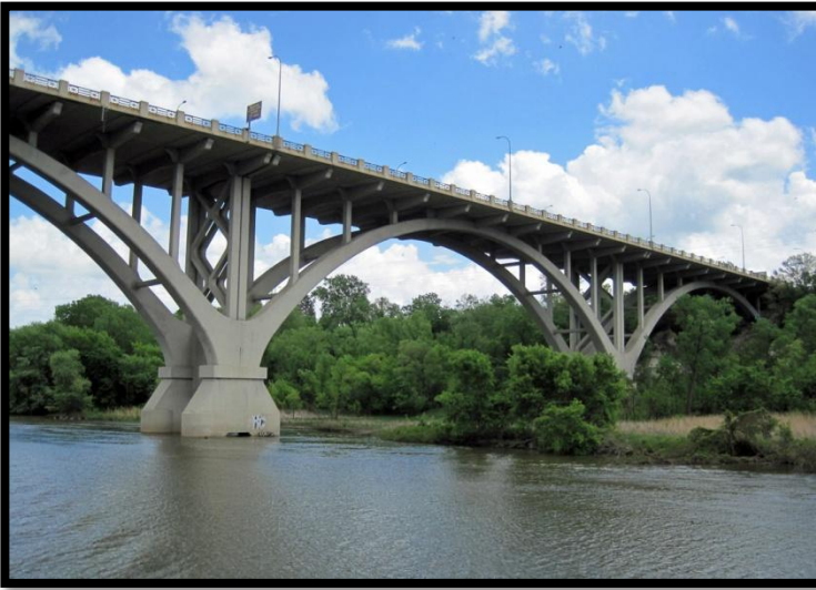
Mendota Bridge opened on November 8, 1926. At the time, it was the longest continuous concrete-arch bridge in the world. For more pictures of the Twin City Bridge during the SIA tour visit Nathan Holth's website Twin Cities Area Bridges
