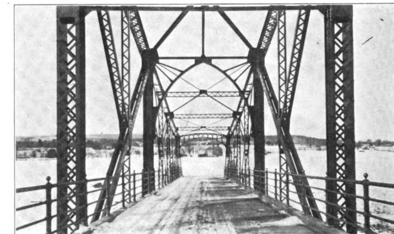
End Span from Near Pier.
