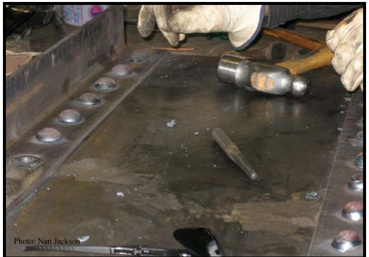
Inspection of rivet removal
