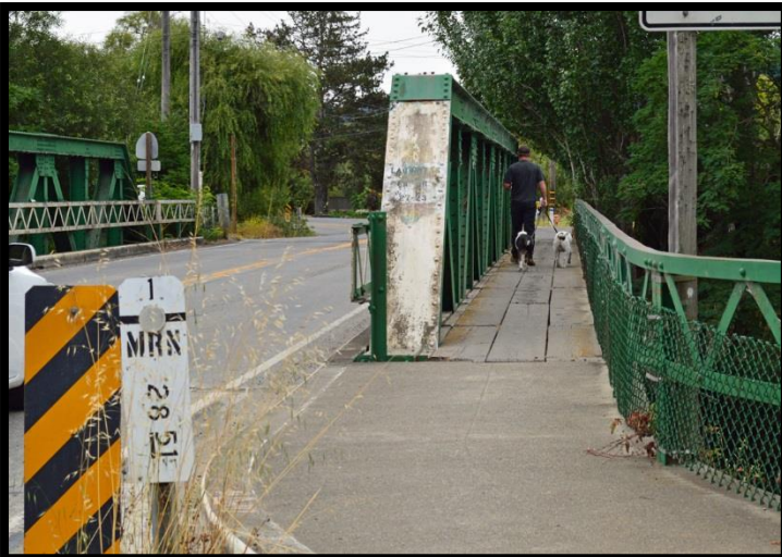
Lagunitas Creek Bridge pedestrian walkway
