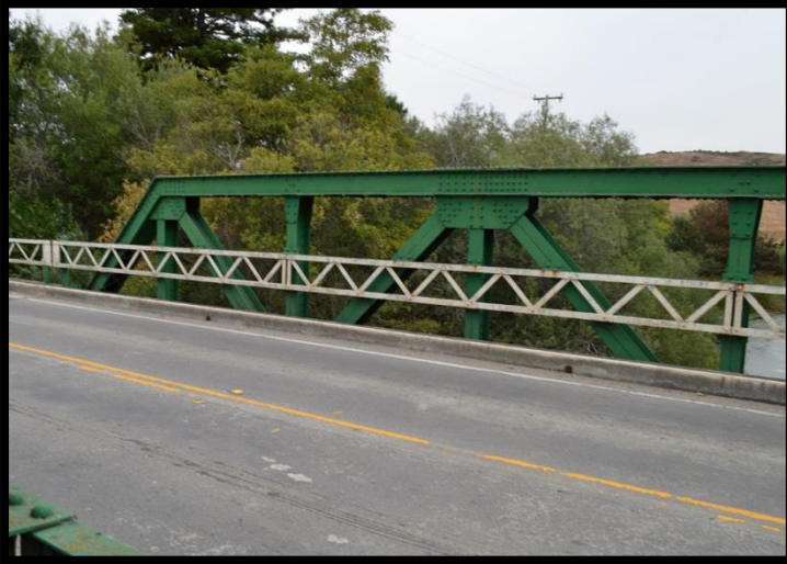
Lagunitas Creek Bridge, a riveted warren pony truss fabricated in 1929
