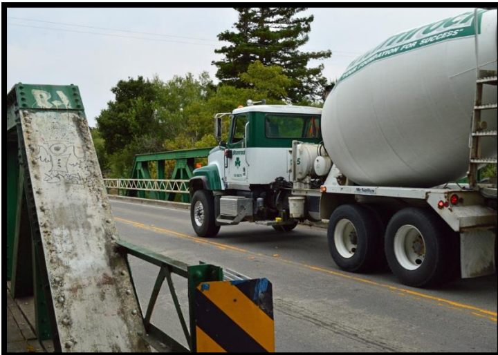
Traffic on the Lagunitas Creek Bridge
