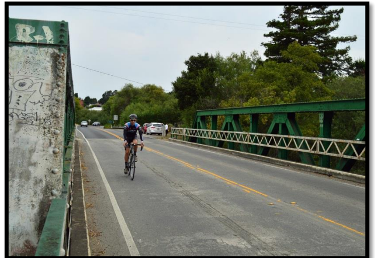
Other traffic on the Lagunitas Creek Bridge
