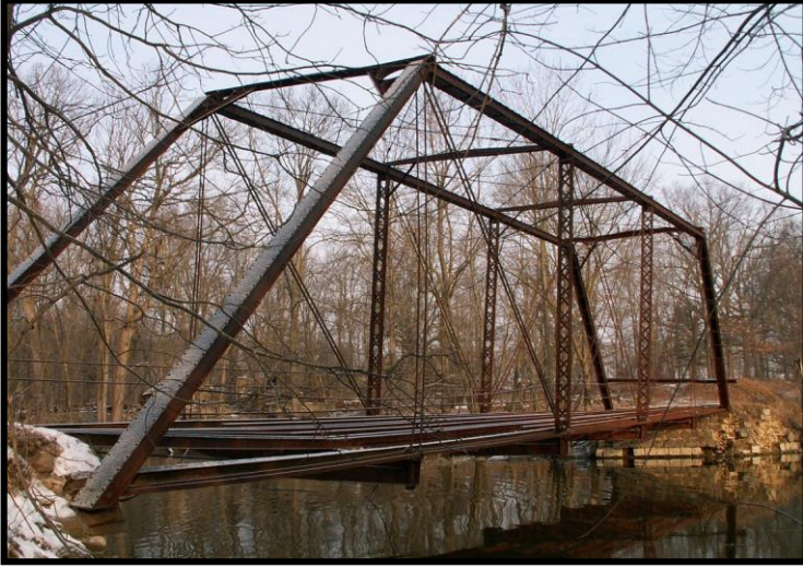
Maple Rapids Road Bridge spanned the Maple Rapids River.
