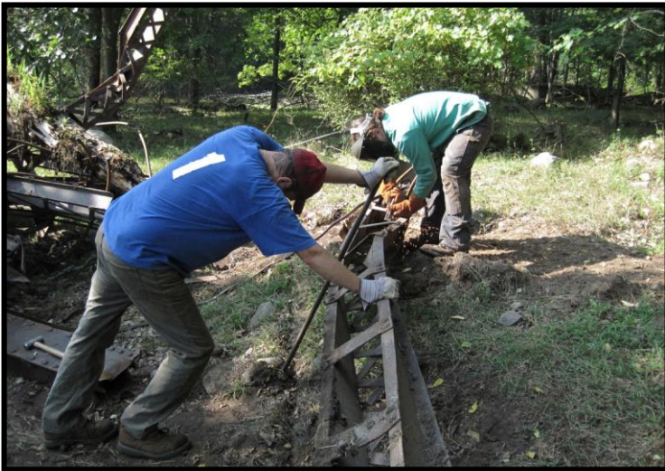
Dace Koenigsnecht, left, assists Dale Franks cutting apart a top chord section.
