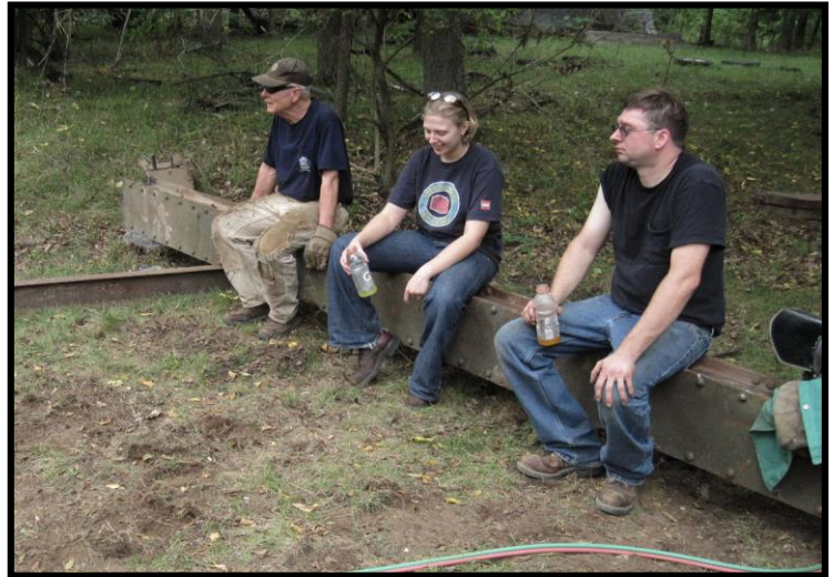
From left to right: Frank Hatfield, Jenna Richelle Lone, and Nate Ellis take a break from dismantling work.
