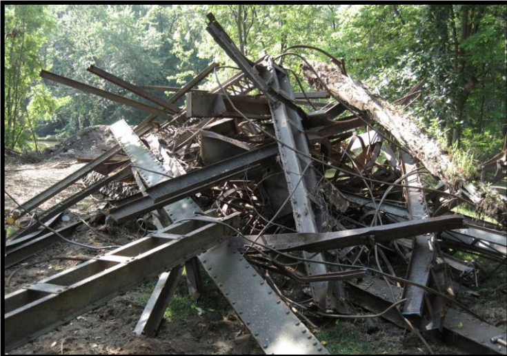
All that was left of the 1888 Maple Rapids Road Bridge after it was pulled from the river was a twisted, bent pile of wrought iron.
