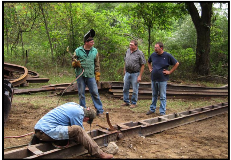
From left to right: Jeff Seelye cuts pin connections, Nate Ellis prepares to cut with the oxygen acetylene torch. Nate L. Ellis and Joe Ellis look on.
