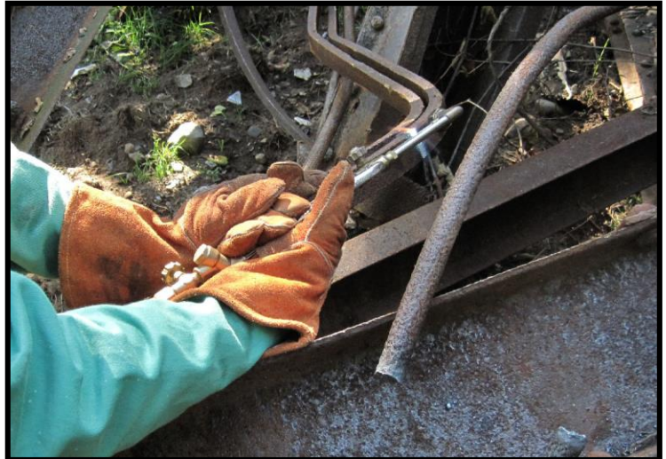
The oxygen acetylene torch was used to dismantle the bent and twisted wrought iron
