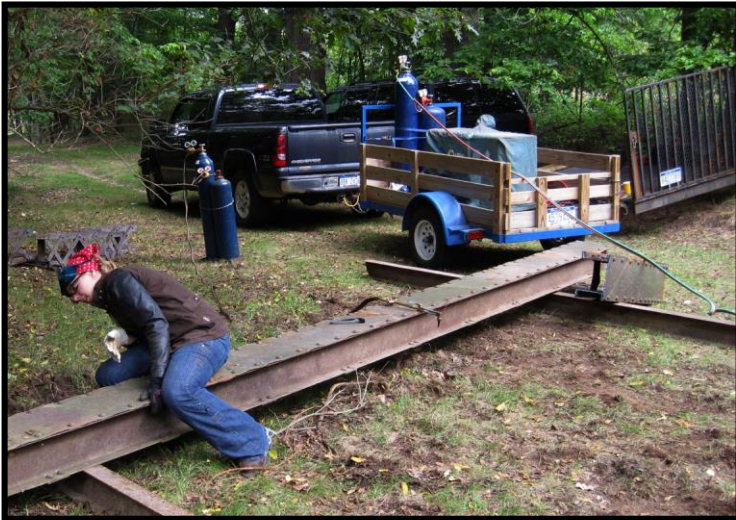
Jenna Richelle Lone, LCC student and LCC welding lab tech, inspects a top chord section of the Maple Rapids Road Bridge for disassembly.
