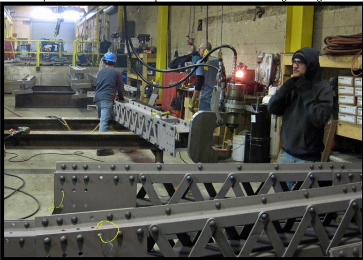
Replicated vertical posts for the Longfellow Bridge Project at Atlantic Bridge & Engineering. (Cianbro Fabrication & Coatings are also replicating rivet assemblies for the Longfellow Bridge Project.)
