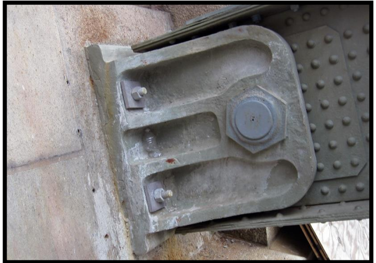
"The ribs are braced transversely by lattice struts and diagonal rods, and are supported on 264 cast steel shoes weighing approximately two tons each" CBC
