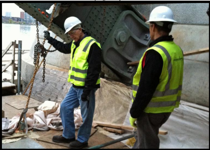
Vern Mesler (Iron & Steel Preservation) and Patrick L. Blais (White/Skanska/Consigli) review rehabilitation work on the Longfellow Bridge
