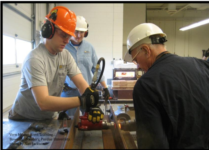
Sherman positions holder-on and Mesler drives rivet. In background is Dave Koppes, Purdue M.S. student, as heater.
