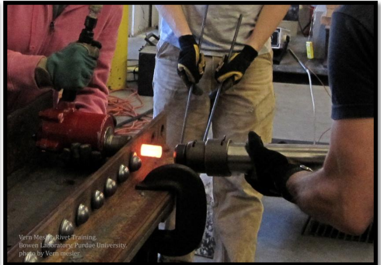
Manufactured head of the heated rivet is held in place with the holder-on.
