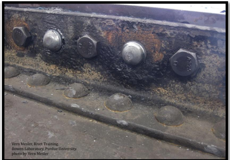
Two new rivets, with more to follow (plate is bolted to angle; new rivets will replace the bolts)
