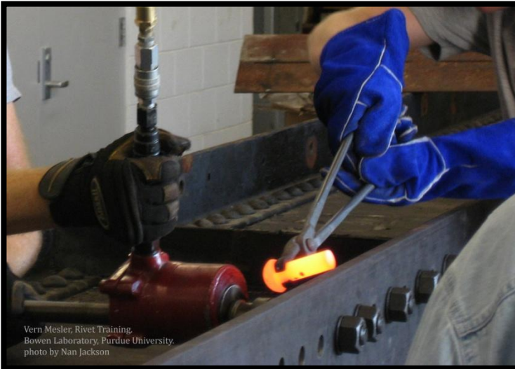
Pneumatic rivet holder-on being positioned to clamp heated rivet in place.
