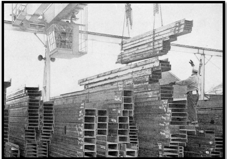
Steel for the Empire State Building was shipped from the Carnegie Steel Company rolling mills in Homestead, PA, and stored at the American Bridge Company and the McClintic-Marshall Company storage yards similar to the storage yard shown in the picture above. (Photo: AISC Textbook of Structural Shop Drafting, vol 1, 1953)
