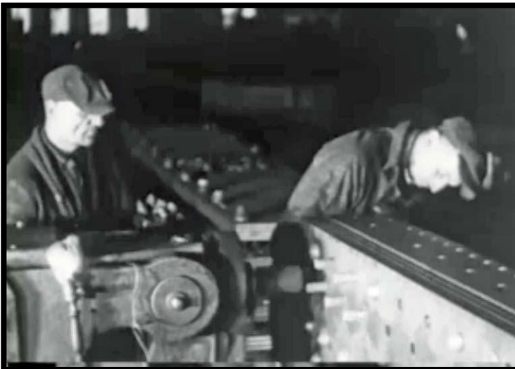
Riveting with a stationary riveter a section for an Empire State Building built-up column section. (Photo: from the film Making A Skyscraper (Steel)-Empire State Bldg. , Prelinger Archives, San Francisco)
