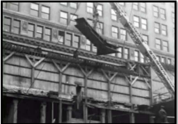
Shop riveted column being set at the Empire State Building construction site. "The Empire State erection plans were complex, and included drawings not usually required, such the erection schedule drawing prepared by Post & McCord." (p 43, Building The Empire State , A 1930s Notebook)
