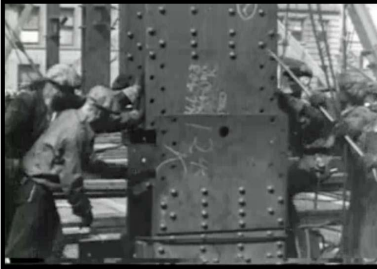
A shop fabricated riveted column is set in place with a derrick crane. (Photo: from the film Making A Skyscraper (Steel)-Empire State Bldg. , Prelinger Archives, San Francisco)
