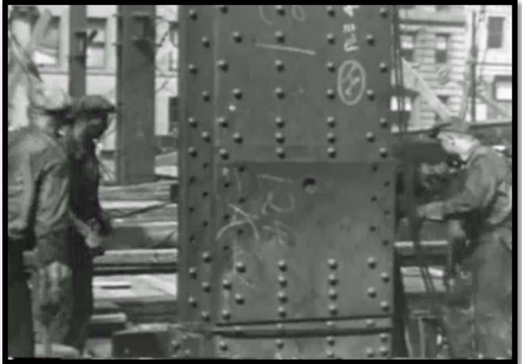
Shop riveted column is set and ready for field riveting. (Photo: from the film Making A Skyscraper (Steel)-Empire State Bldg. , Prelinger Archives, San Francisco)
