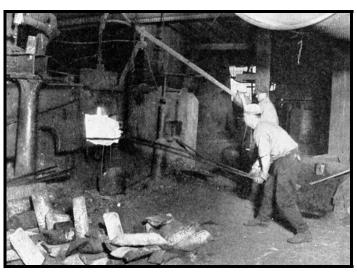
Charging the puddling furnace with pig iron
