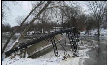
The wrought iron bridge that lay on its side, its bent inclined end post anchored to a tree, is the Parshallburg Bridge built by the Wrought Iron Bridge Co. of Canton, Ohio, 1889.
