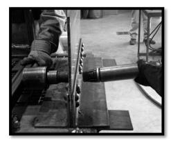
Hot riveting for replacing historic rivets and replication of historic riveted structures.
