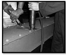
Pack rust removal, heating and hammering
