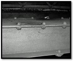
Restoration of metal damaged by pack rust
