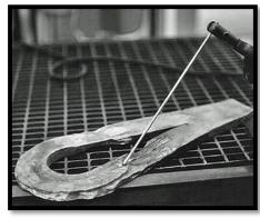
Arc welding section-loss in wrought iron and historic steels
