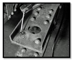
Removing rivets with the Air Carbon Arc process for rivet restoration
