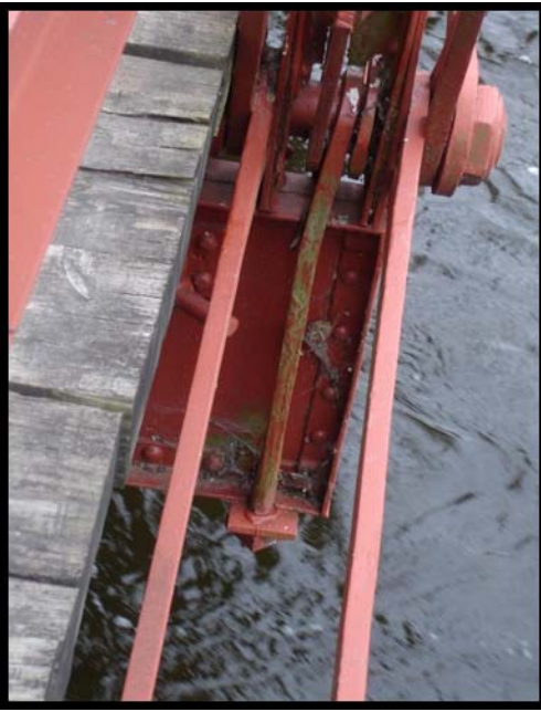
Photo 6: Riveted wrought iron floor beam, East Delhi Bridge, Washtenaw County, Michigan
