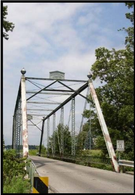
Photo 1: TR 241 Bridge in 2008
