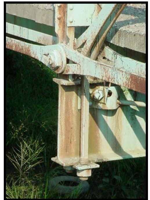
Photo 5: I-beam (American Standard Beam) Speaker Road Bridge, St Clair County, Michigan
