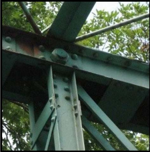
Photo 13: TR 241 Bridge top chord and vertical pin connection with recessed nut
