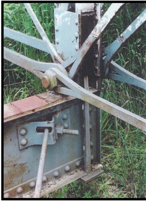
Photo 7: Riveted wrought iron floor beam, Bell Road Bridge, Washtenaw County, Michigan (with good view of eye-bar above the floor beam)
