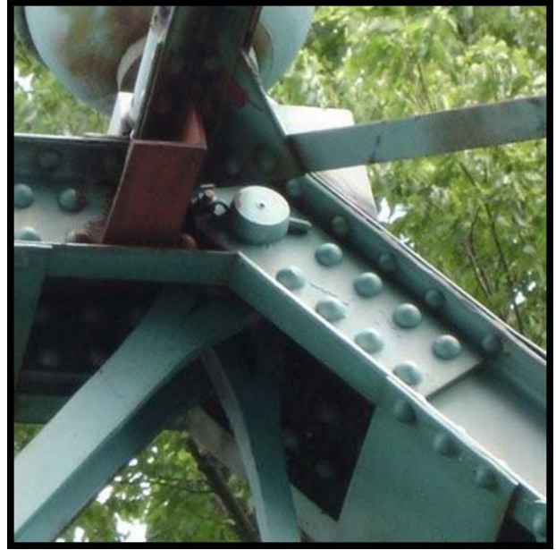
Photo 14: TR 241 Bridge top chord and inclined end post pin connection with cotter key
