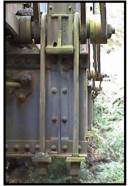
Photo 8: Riveted wrought iron floor beam, Haupt Creek Bridge, Sonoma County, California
