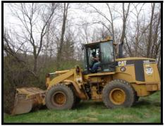
Del Sears guides the County's Caterpillar 966E front end loader along the top of the west abutment site, clearing the brush and trees. Occasionally the heavy front tires would sink deep in the loose sandy soil, but a few quick moves with the 5-yard bucket and Sears has the front end loader clear and resumes grubbing.
