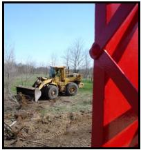
With an experienced hand Matthews pushes down trees with the front end loader's bucket, then picks each downed tree slightly off the ground with the bucket and shakes the dirt free from the tree roots. Each tree is then stacked in a pile, then that pile is lifted high and dumped on the growing accumulation of trees and brush.
