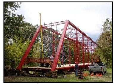
On September 29<sup>th</sup> two inclined end posts and portals were set in place. After pinning and bolting everything in place the gin pole and scaffolding will be moved to the other end of the bridge to finish the last two panels of the Charlotte Highway Bridge.
