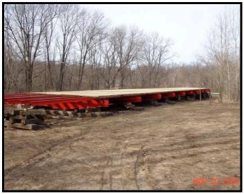
During the spring of this year Conklin and Denniston began installing the wood deck on the replicated floor beams of the Charlotte Highway Bridge in preparation for putting up the trusses. The gin pole was also being fabricated at this time with the help of Frank Hatfield, P.E. Professor Emeritus, Civil and Environmental Engineering, Michigan State University. On May 24<sup>th</sup> it was placed on the deck.
