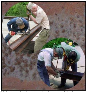
Volunteers riveting a top chord section of the Stearns Truss bridge (top picture) and removing pack rust (bottom picture) Photo by author
