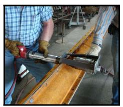
Jeff Gawell and Neil Campbell hammer a rivet in a restored Phoenix column from the Zoarville Station Bridge. Gawell and Campbell fabricated a fixture (right) that holds in place a holder-on that keeps the hot rivet firmly in place as the rivet hammer drives the rivet. Photo by author
