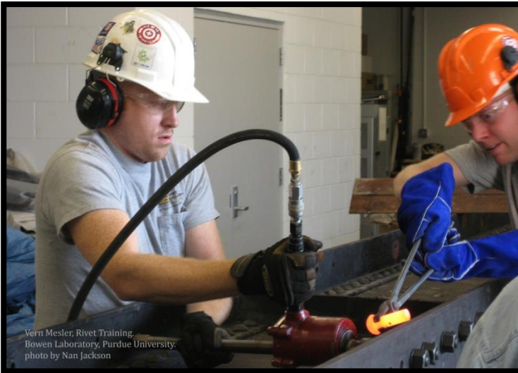
Hebdon positions holder-on with extension bar; Sherman inserts heated rivet.
