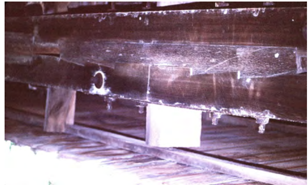
West Union Bridge, Parke County
