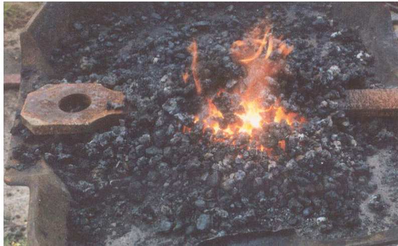
Figure C.3 Heating of Eyebar from Bell Ford Bridge Prior to Straightening
