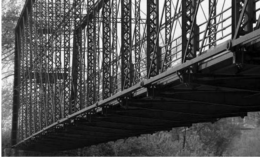
Figure 5.3 Picture of Bottom Chord of Laughery Creek Bridge, Spanning Laughery Creek, Aurora vicinity, Dearborn County, IN (Historic American Buildings Survey/Historic American Engineering Record)
