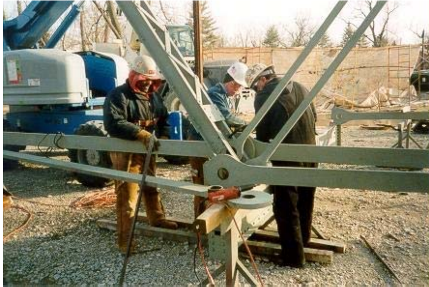
Figure 5.11 Reassembling a Pin Connection After Members Have Been Sand Blasted and Repainted During A Rehabilitation of a Bridge in Plainfield, IN
