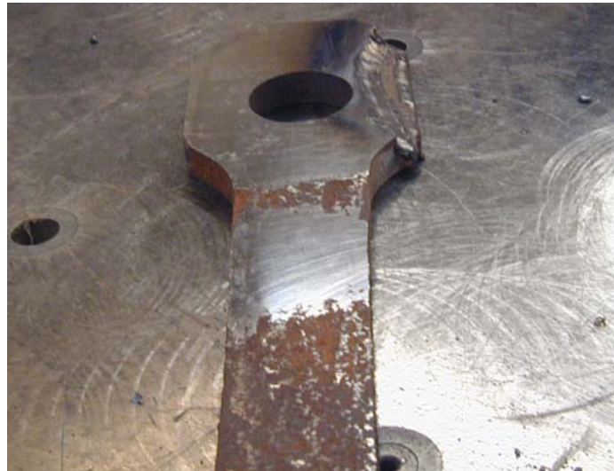
Figure C.26 Eyebar End Connection A after Half of Filler Weld Repair Completed
