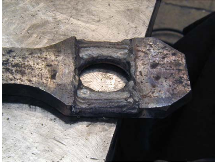
Figure C.27 Eyebar End Connection B after Half of Filler Weld Repair Completed
