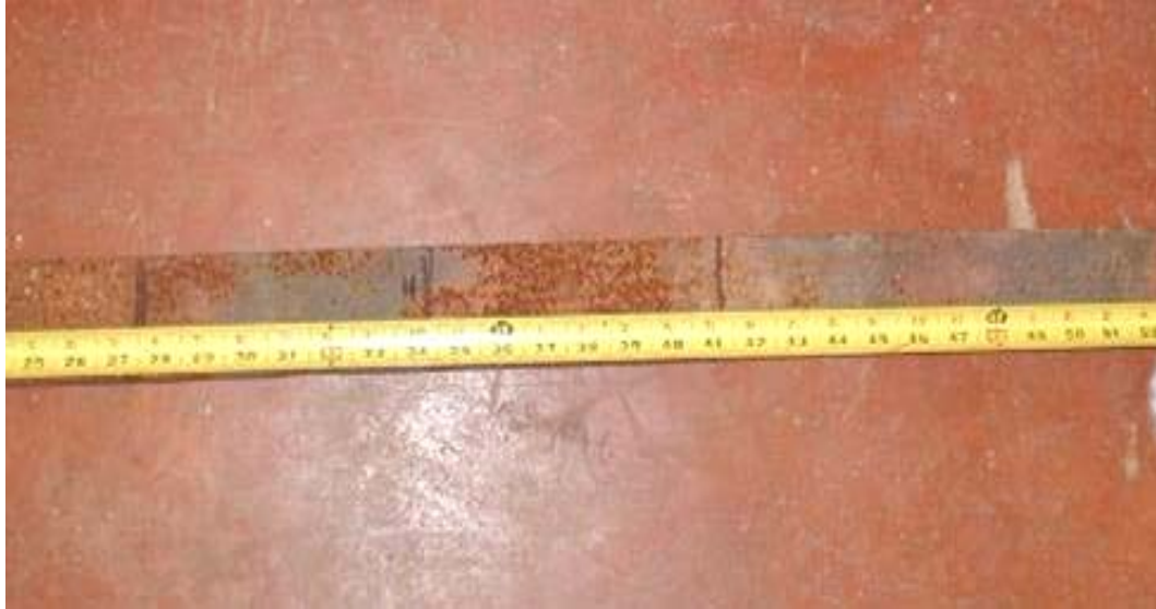
Figure 3.7 Heated Areas in Blue on Eyebar 2
