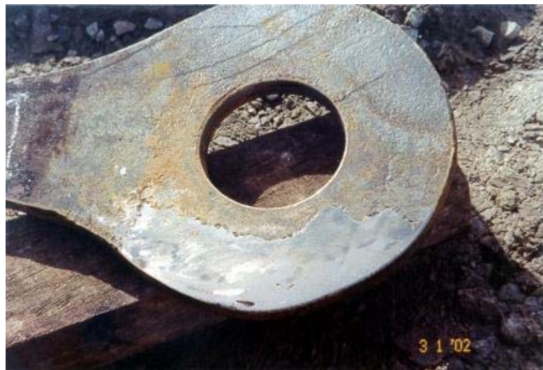
Figure 5.10 Filler Weld Completed in the Field to Repair Corroded Eyebar Connection
