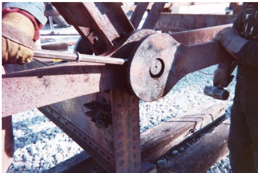
Figure 5.7 Using Force After Using Heat to Disassemble A Pin Connection During a Rehabilitation of a Wrought Iron Bridge In Plainfield, IN.
