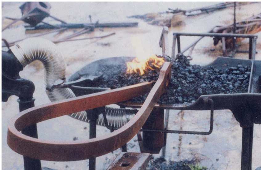
Figure 5.14 Heating and Straightening Damaged Members of the Bell Ford Bridge
