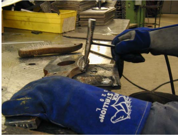
Figure C.25 Chisel Hammer to Remove Surface Slag of Filler Weld in Eyebar End Connection Repair
