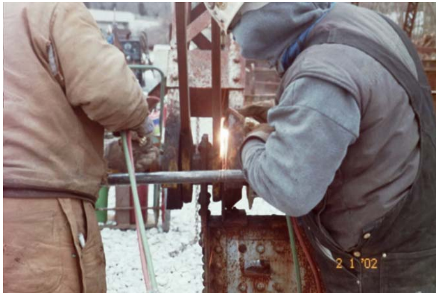
Figure 5.6 Using Heat to Help Remove a Pin During a Rehabilitation of a Bridge In Plainfield, IN.
